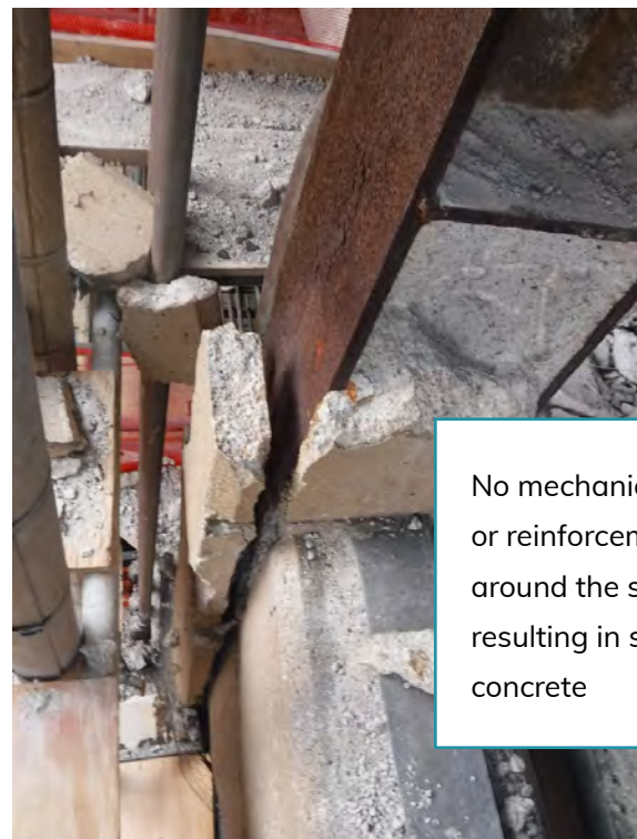
Figure 2: Concrete Spalling
