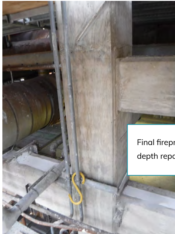
Figure 4: Final Fireproofing
