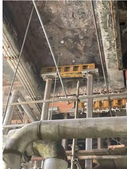
Photo of Deteriorated Area and Shoring System
