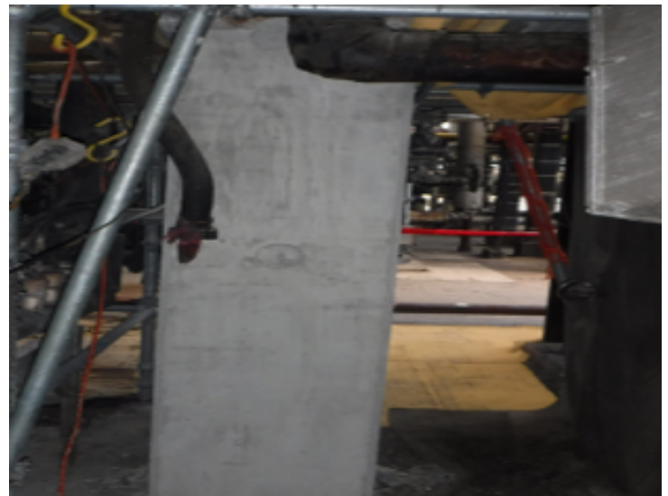
Full concrete repair completed
