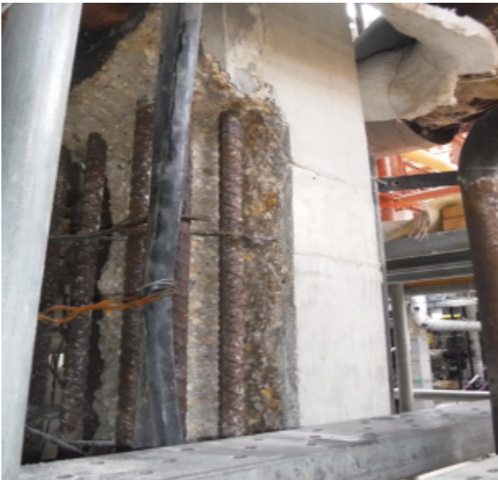
Partially concrete repair in progress
