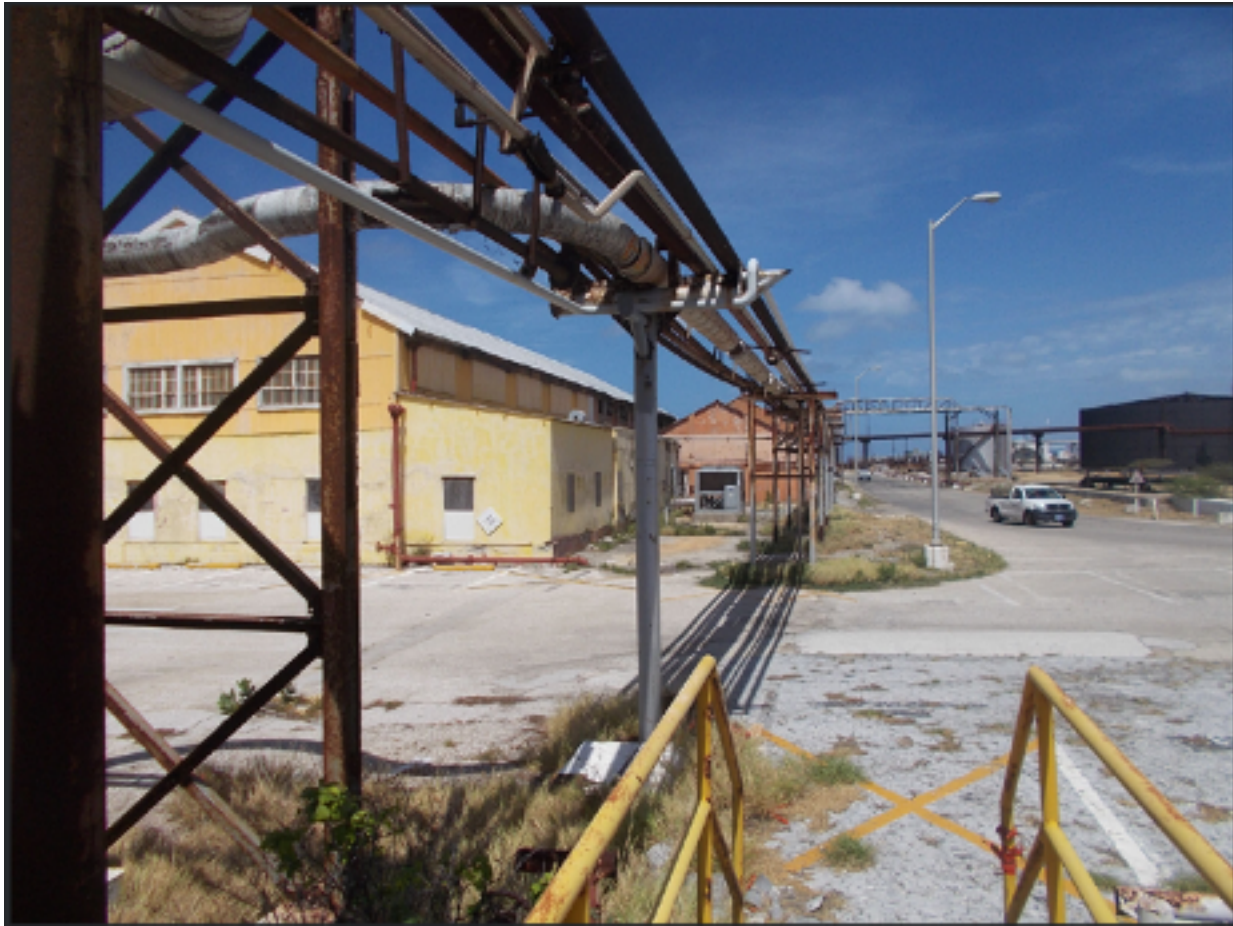
View of Pipe Bridge as Found
