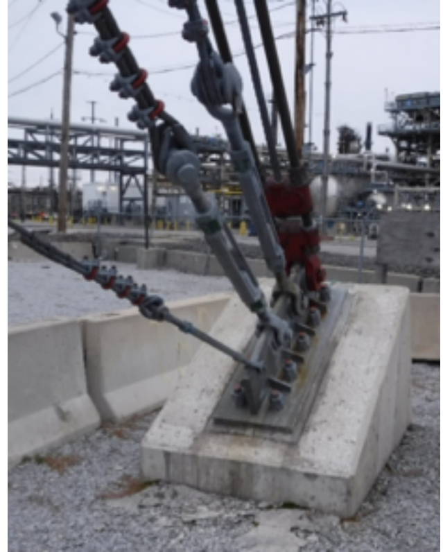
Typical Guy Wire Anchorage
