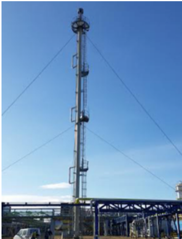
Typical Guyed Flare Tower
