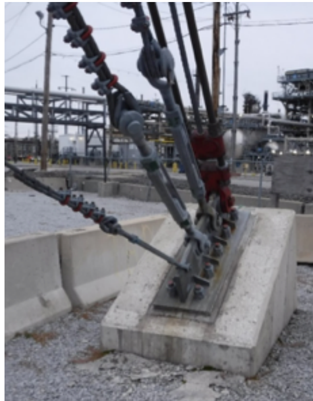
Typical Guy Wire Anchorage
