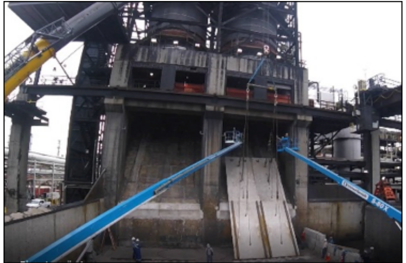
View of Wear Plate Being Installed
