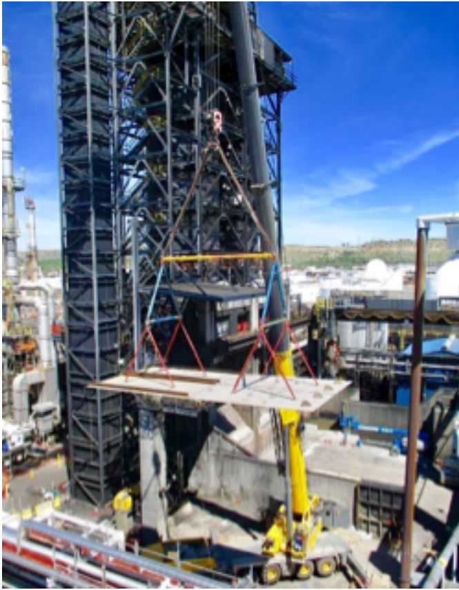
View of Wear Plate Being Lifted
