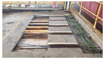
Fig. 4: Placement of new PT anchors
