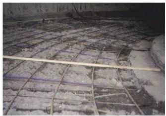
Fig. 3: Demolished ramp slab surface with supplemental post-tension reinforcing installed throughout central cylinder
