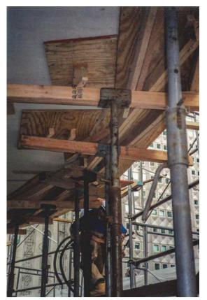
Fig. 6: Slab edge formwork and shoring
