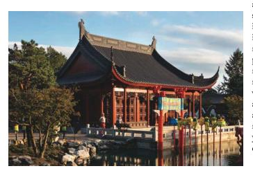
plus the ability to withstand Quebéc's harsh winter weather conditions were key selection criteria. The project included reconstructing areas of the roofs and garden walls, repairing and setting terracotta tiles on the roofs and providing a protective coating.
