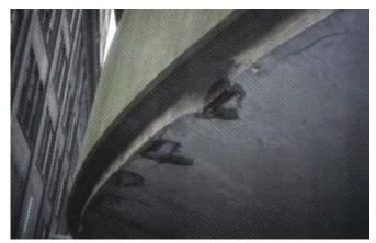
Fig. 2: Original slab edge deterioration
