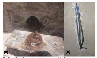
Fig. 3: (a) Corroded post-tension anchor, and (b) Ruptured tendon
