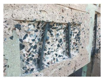
Fig. 5: Hand-applied repair
