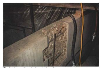
Fig. 8: Knee wall vertical repair demolition
