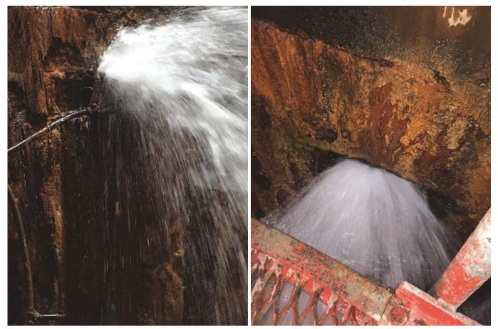
Fig. 2: Major water penetration points were blasting masses of water 12 in (300 mm) wide across the 23 ft (7 m) diameter of the shaft. The extreme pressure of the water was causing damage to the shaft structure and made the repair a very dangerous project.
