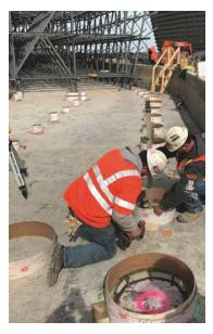
Accordingly, an extensive restoration and rebuild of the cooling tower was planned during a 6.5 week shutdown in May 2017. Rebuilding the cooling tower required the following steps: Demolition of the exterior
