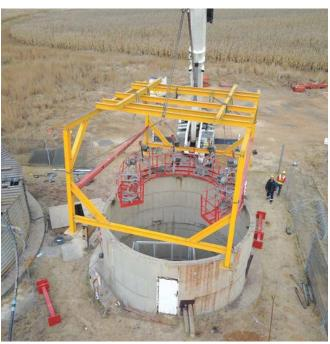
Fig. 3: Access to the shaft was a huge safety and logistical concern. The access specialists were able to supply a custom-built cradle to lower workers into the shaft. This cradle was anchored to the sides of the shaft to ensure no movement during the high-pressure cleaning and sandblasting.
