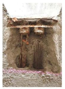
Fig. 3: Many beams were observed to have completely corroded through tendons
